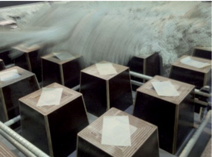
Individual formwork construction
