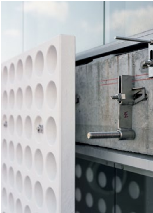
550 m² fibreC 3D elements with a thickness of 7 cm are cladding the Lontoonkatu 9 project in Helsinki, designed by Kirsi Korhonen and Mika Penttinen Architects. The entire facade was divided into 16 different types of panels with lenghts up to 3.8 m. More than 400 concrete elements with faced concrete quality on both sides offer an interesting view from inside of the building.
