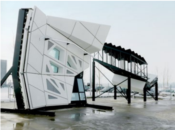
Combination of fibreC 3D and extruded fibreC elements
