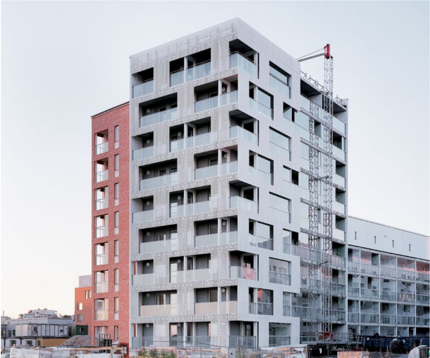
550 m² fibreC 3D elements with a thickness of 7 cm are cladding the Lontoonkatu 9 project in Helsinki, designed by Kirsi Korhonen and Mika Penttinen Architects. The entire facade was divided into 16 different types of panels with lenghts up to 3.8 m. More than 400 concrete elements with faced concrete quality on both sides offer an interesting view from inside of the building.
